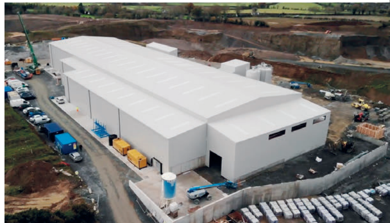
Kilsaran Precast in Kilcullen, County Kildare is the most modern and automated carousel plant in Ireland.
