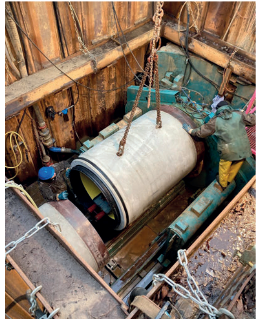
Space is usually at a premium in pipe jacking operations. This makes the Perfect Jacking Pipe even more advantageous, as a complete, corrosion-protected pipe system is created as soon as the next pipe is inserted.
