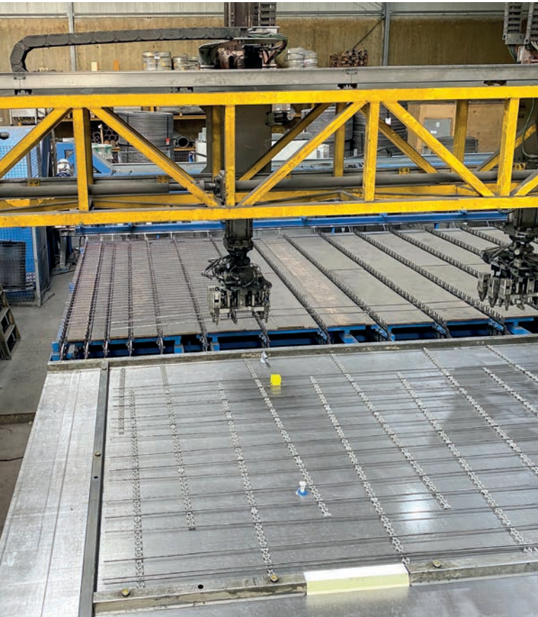
The 6-fold EPT laying grab works fully automatically according to CAD-CAM specifications.
