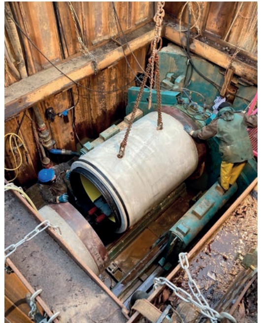
Space is usually at a premium in pipe jacking operations. This makes the Perfect Jacking Pipe even more advantageous, as a complete, corrosion-protected pipe system is created as soon as the next pipe is inserted.
