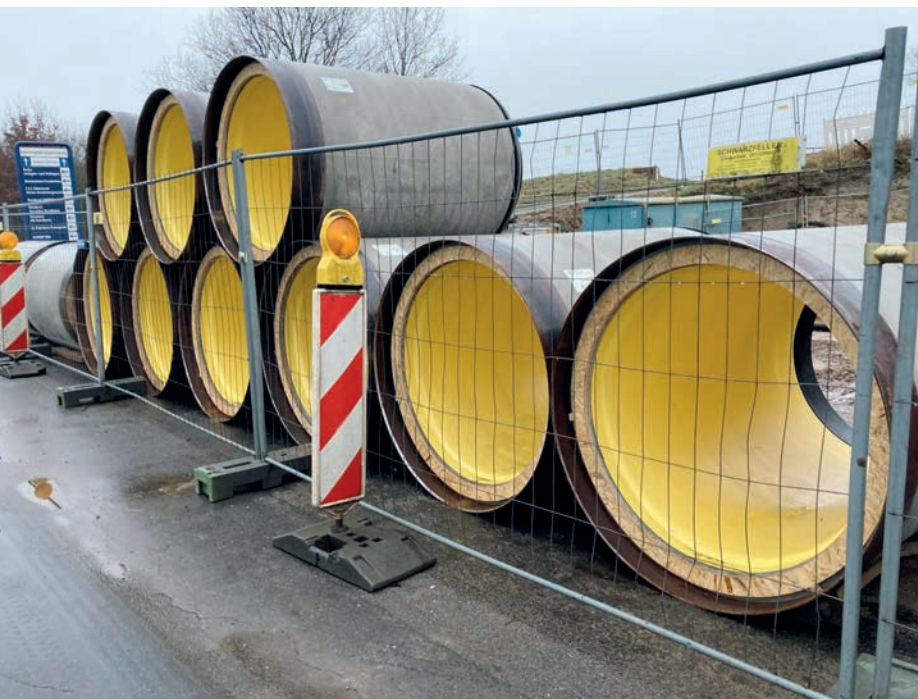
Typical Perfect Pipe construction site store (Haren, Deutschland). The first Perfect Pipe DN 1200 jacking pipes in Germany were installed here in 2021.
