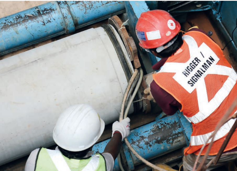
Installation of Perfect Pipe jacking pipes in the first project of its kind implemented in Singapore—this was reported on in CPI 2/2016.
