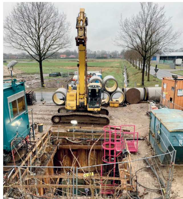
Typical Perfect Pipe construction site store (Haren, Deutschland). The first Perfect Pipe DN 1200 jacking pipes in Germany were installed here in 2021.
