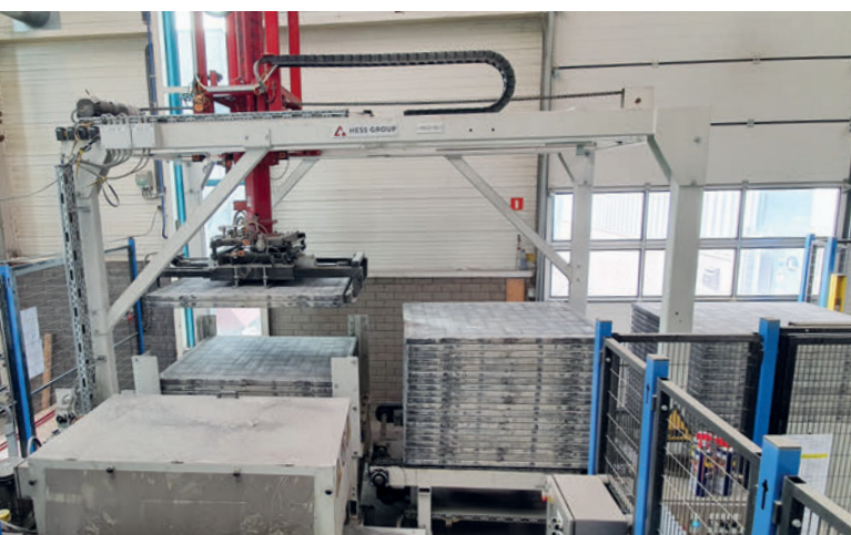
Production board buffer conveyor with destacking crane and board hopper
