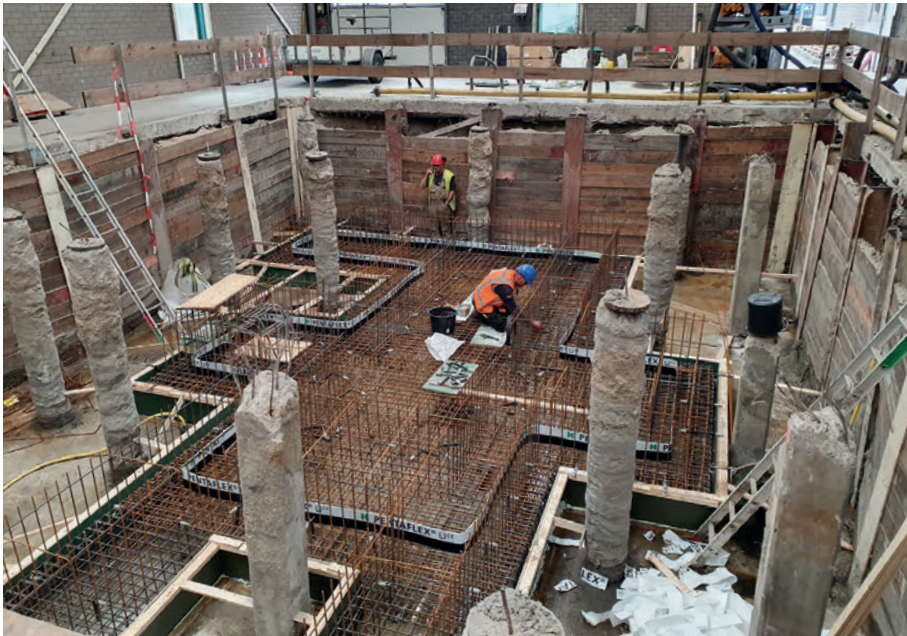
Machine pit under construction before pouring of concrete
