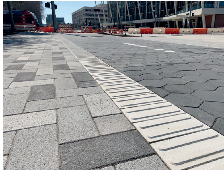
Bagby Street: Stone installation pedestrian and bicycle area
