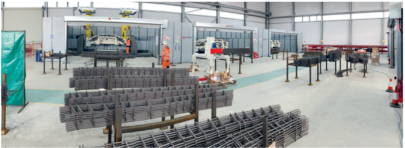
The prefabricated ladders are welded together with the reinforcement meshes by the welding robots (visible in the background) to form the finished cage for tunnel elements.
