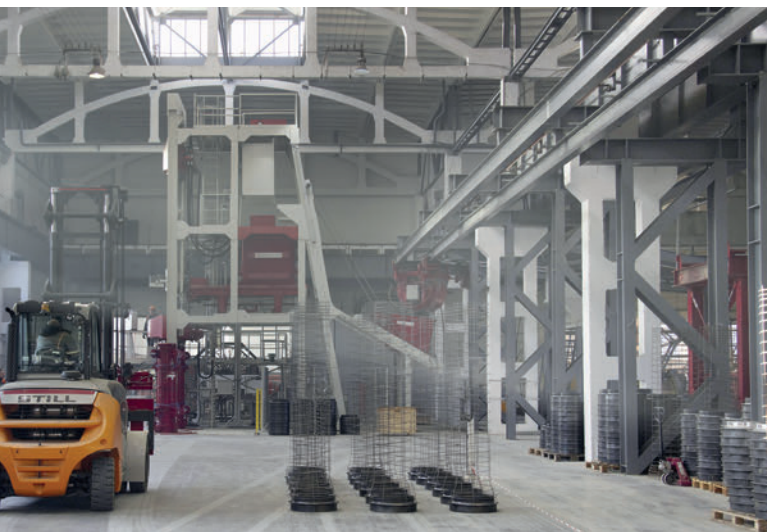
Concrete pipe production with the Radial Press at the Minskmetrostroy concrete plant
