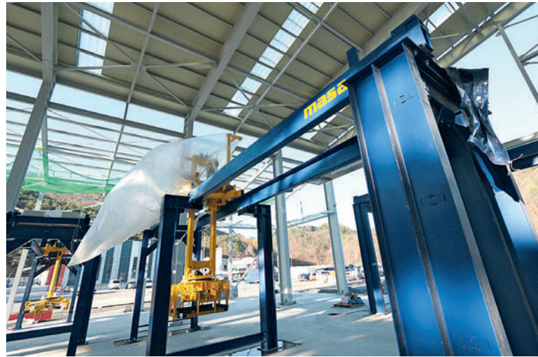
The new plant in Danyang is taking shape step by step.
