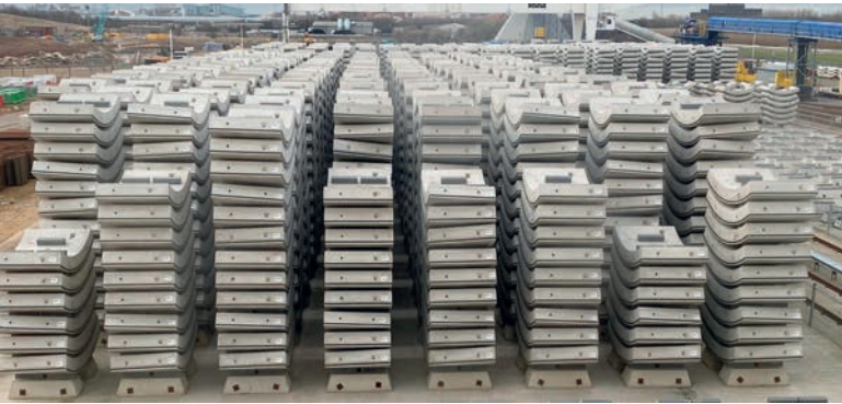
Temporary storage of the lining segments - the concreted prefabricated elements for the outer shell of the tunnel
