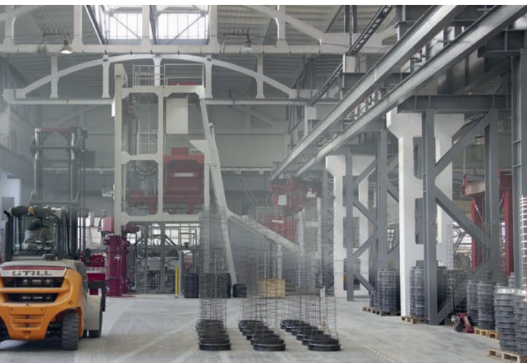
Concrete pipe production with the Radial Press at the Minskmetrostroy concrete plant
