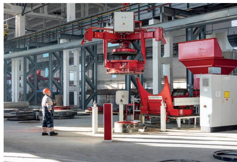
Atlas 150/150 - Manhole cover slab production
