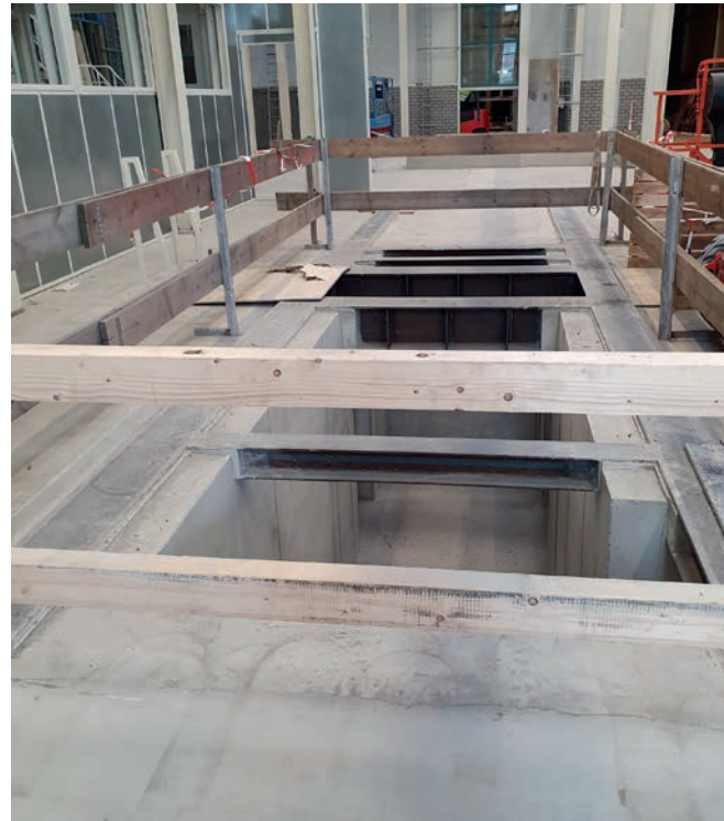
Machine foundation shortly before installation
