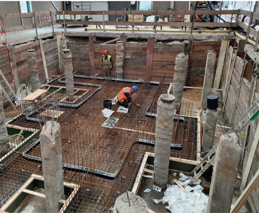
Machine pit under construction before pouring of concrete
