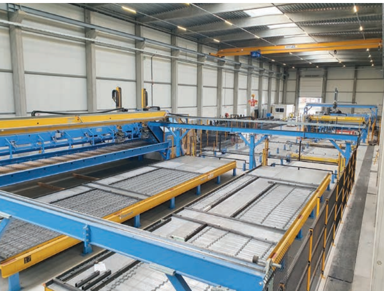
Extended view of the plant with the automatic wire processing units as well as the fully automatic shuttering robot including a pallet cleaning device.
