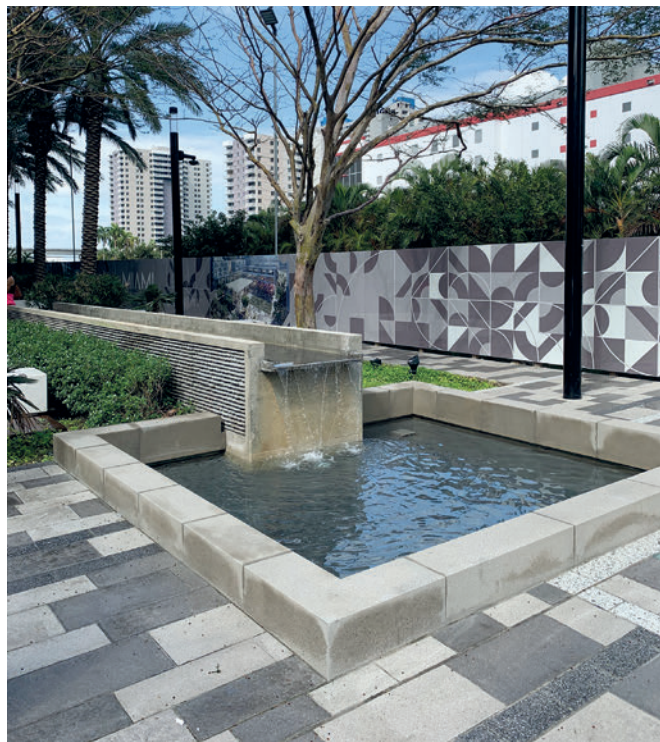
Laying Wausau pavers
