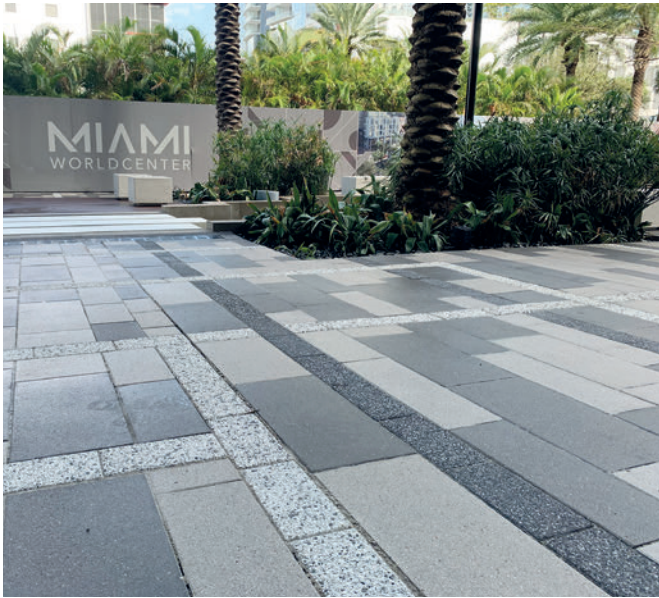
Laying Wausau pavers
