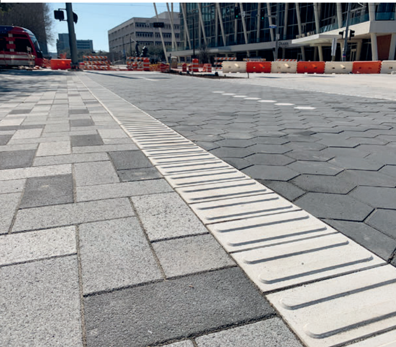
Bagby Street: Stone installation pedestrian and bicycle area
