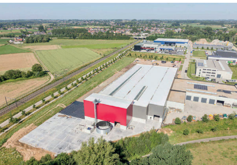
The new production facility in Aalst is fully operational for production and equipped with the latest technology.
