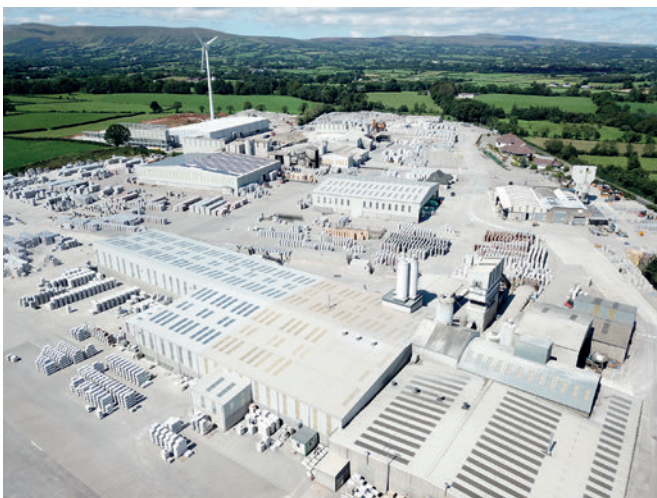
The plant site in Tobermore - the new production hall IV can be seen in the background below the wind turbine.
