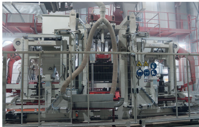
The Hess RH 1500-4 MVA concrete block machine is the heart of the production plant.
