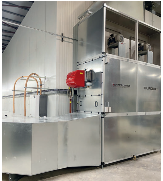
The ideal climate in the individual chambers is ensured by the latest-generation Quadrix Ultra concrete curing system from manufacturer Kraft Curing Systems.
