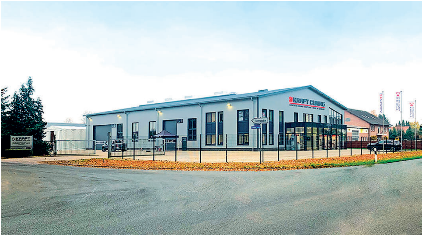
New Kraft Curing Systems GmbH production hall and office building
