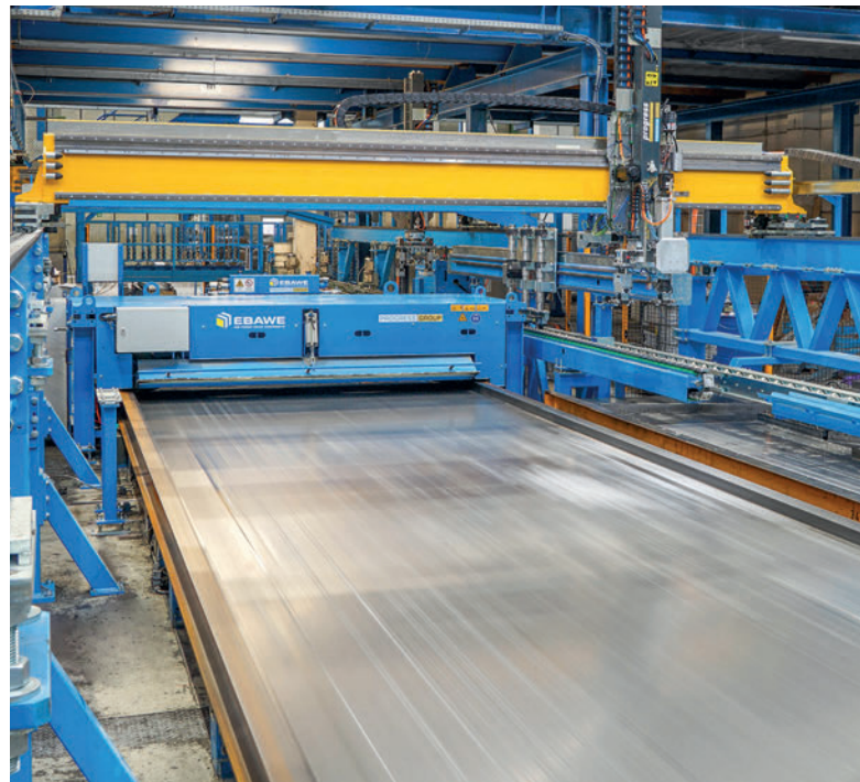
The Ebawe pallet cleaner is also part of the new shuttering robot.
