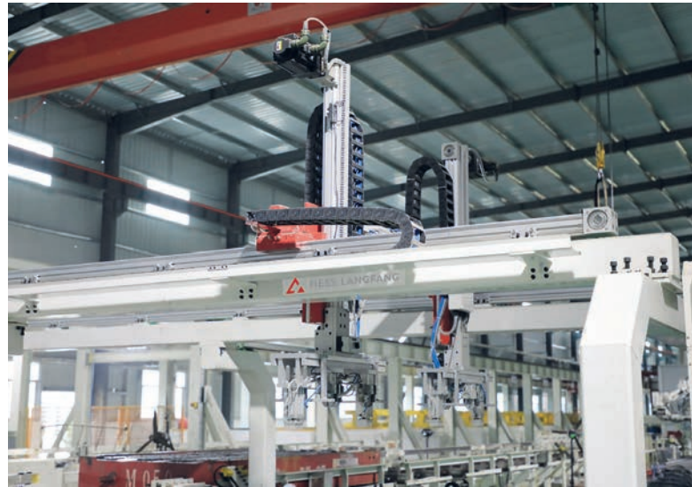
Figure 8: Automated railway sleeper steel reinforcement installation station
