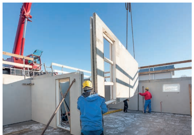
Schwörer cellar assembly – the basis of Schwörer prefabricated houses.
