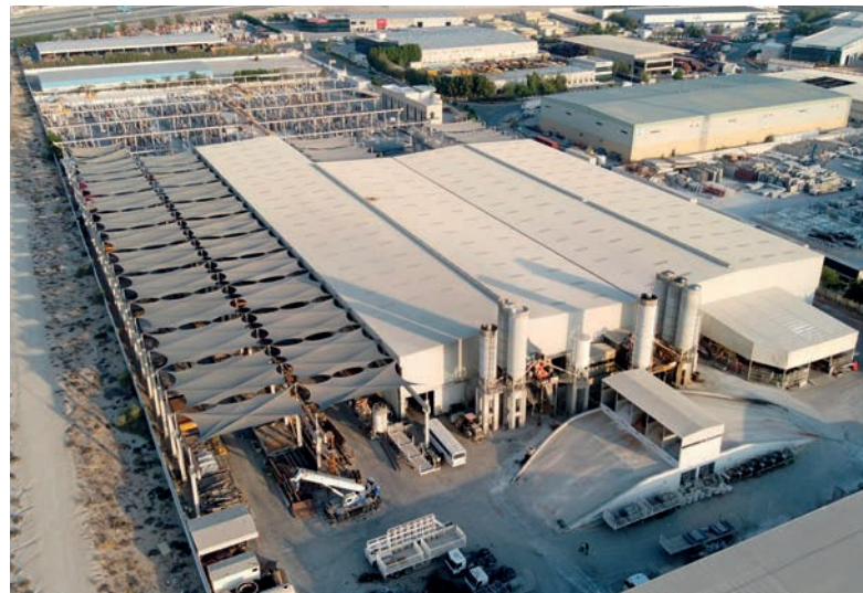
View of Hard Precast's company site in Dubai and the stored precast concrete parts.
