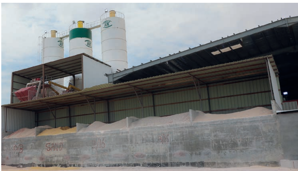
Production site of Riyadh Kingdom Concrete Products Al Ahsa
