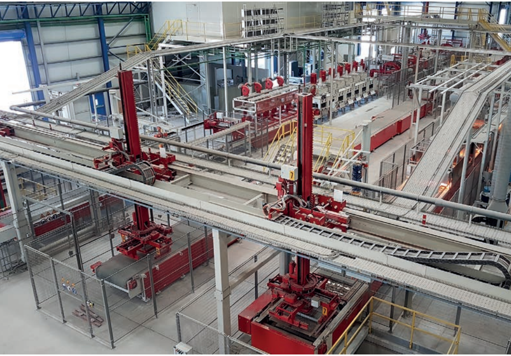
Figure 2: SR Schindler material handling system „Made in Germany“
