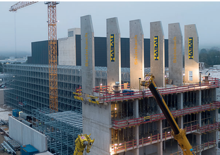
Assembling special precast concrete elements at a construction site
