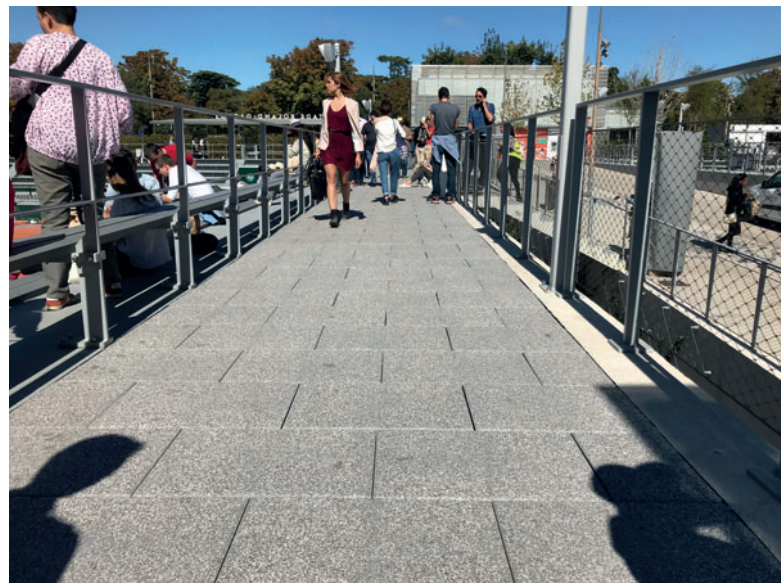
Laying in pedestrian areas
