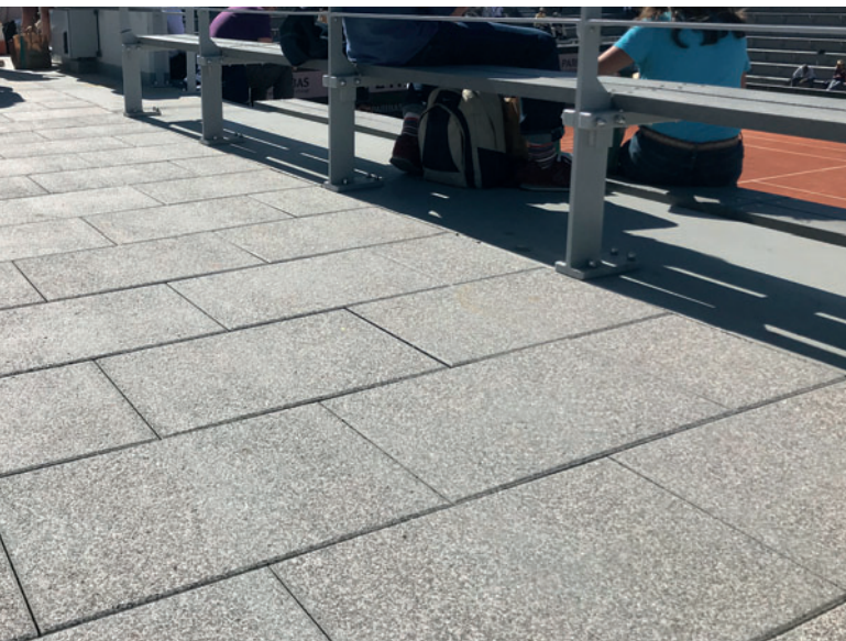
Detail view of concrete slabs
