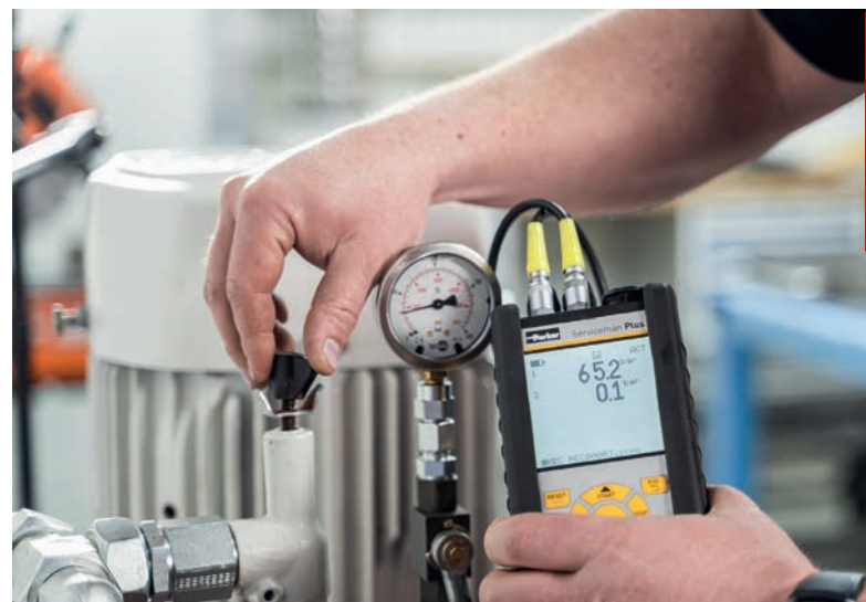
Checking the system pressure
