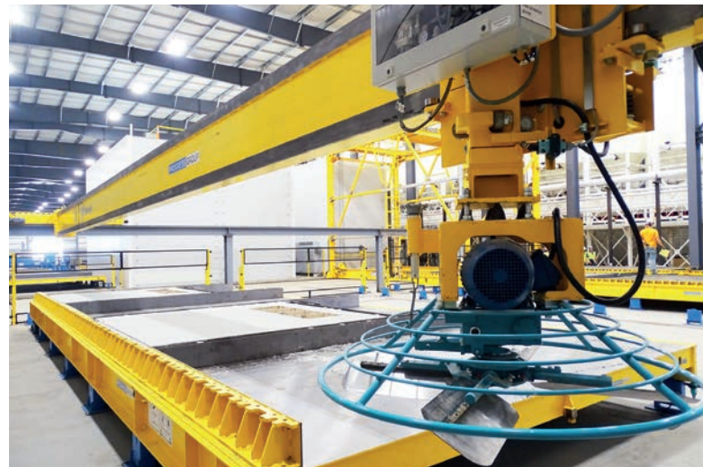
A power trowel is used for fine smoothing, resulting in a very finely smoothed, paintable concrete surface that does not require any subsequent post-processing.
