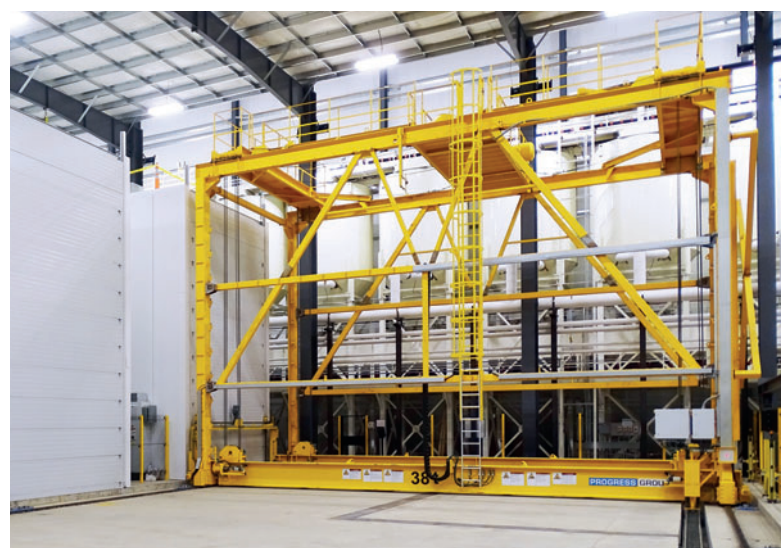
The pallet stacker serves the two racks and stores and retrieves the pallets with the freshly concreted solid wall elements.
