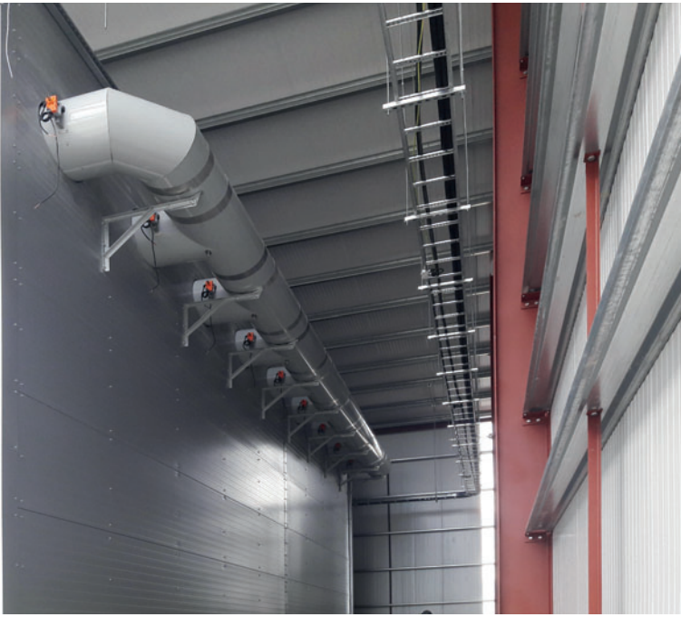
Precise control: each individual chamber has its own vapor supply using high-quality stainless-steel components and steel jacketed mineral wool insulation for a clean, durable and economical solution.
