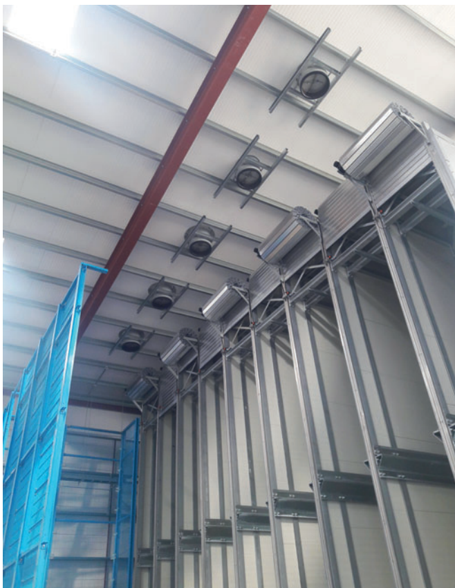
Nine independently controllable individual chambers form the new curing system for concrete slabs from the radial press and allow Kilsaran maximum flexibility in production.
