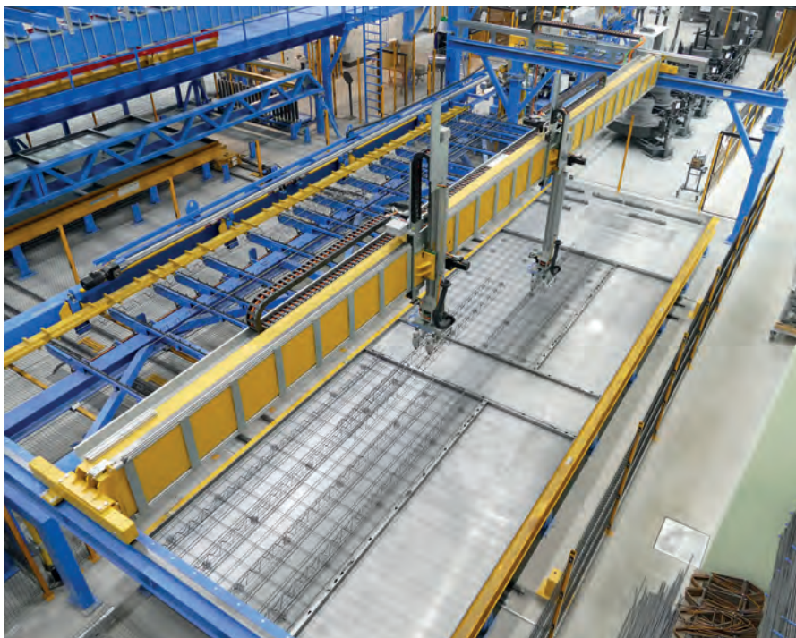
A multi-axis linear robot rounds off the automated reinforcement area in Eder's new plant.
