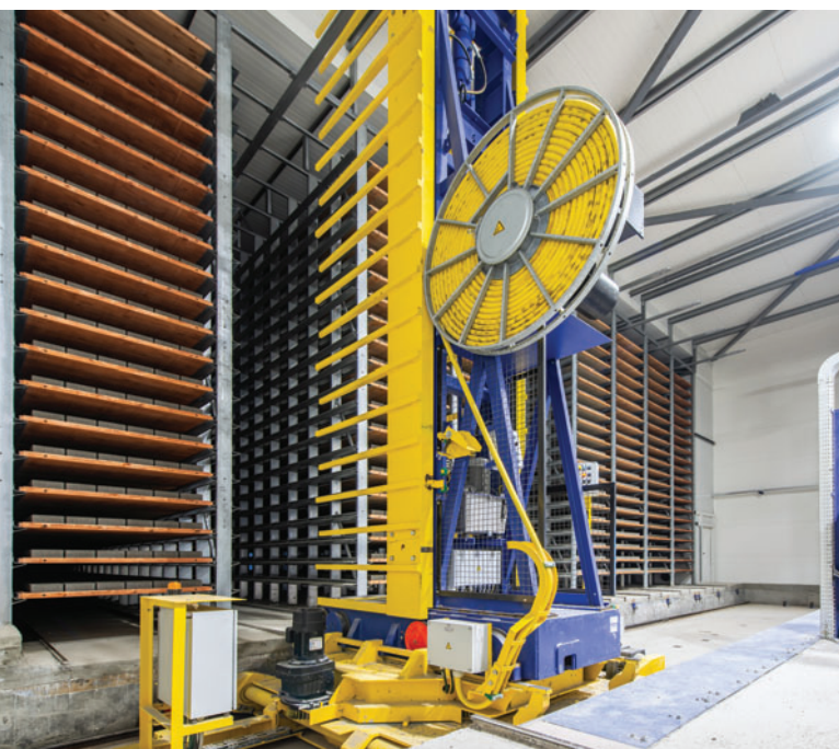
Storage and retrieval of the concrete blocks in the curing chambers
