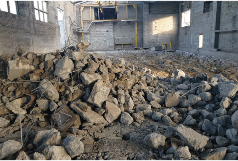
The demolition work progresses
