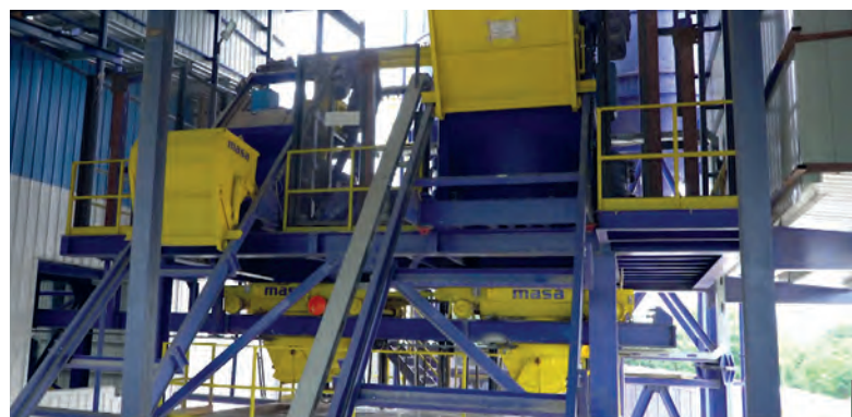
Aggregate hoists to the Masa concrete mixers
