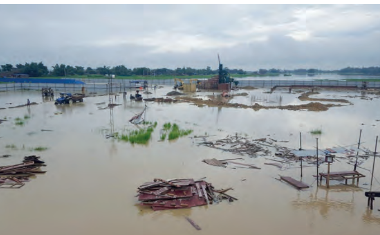
Flooding of the site after heavy monsoon rains
