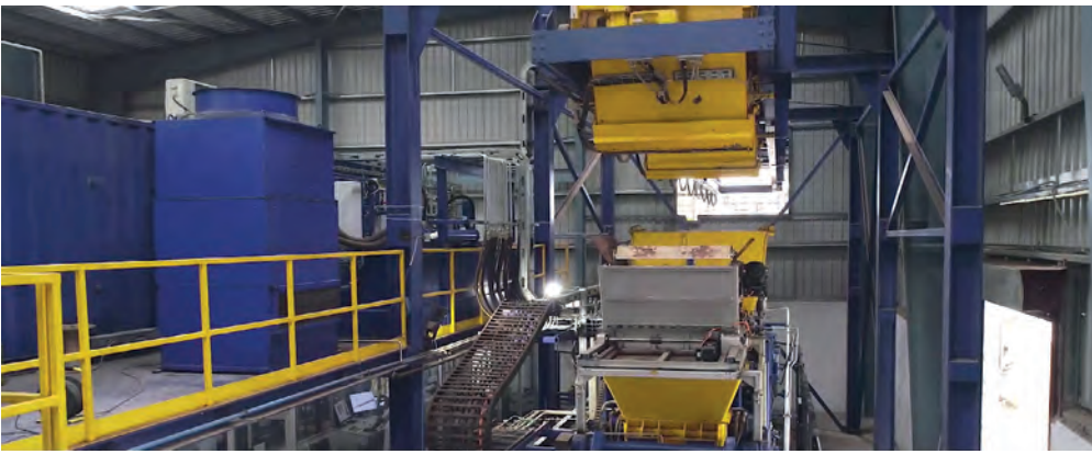
Concrete transport via bucket conveyor to the concrete block making machine
