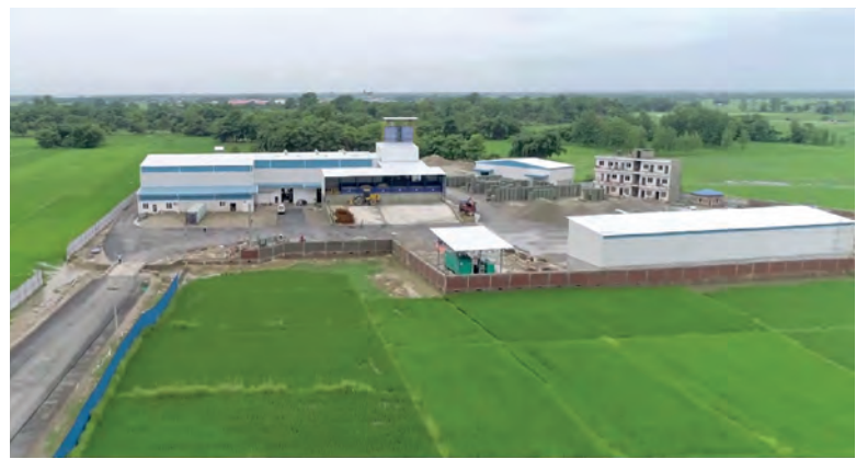
Since June 2018, high-quality concrete blocks and pavers are produced in Ramgram
