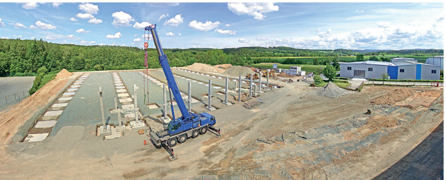
Kobra builds four new production halls
