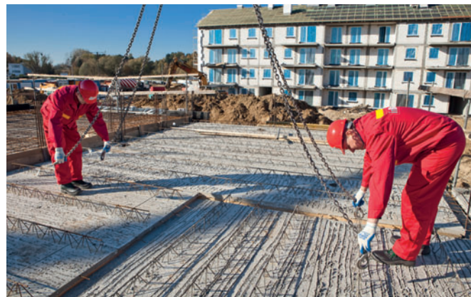
Filigree slabs allow for quick and tailor-made floor slab production and installation.
