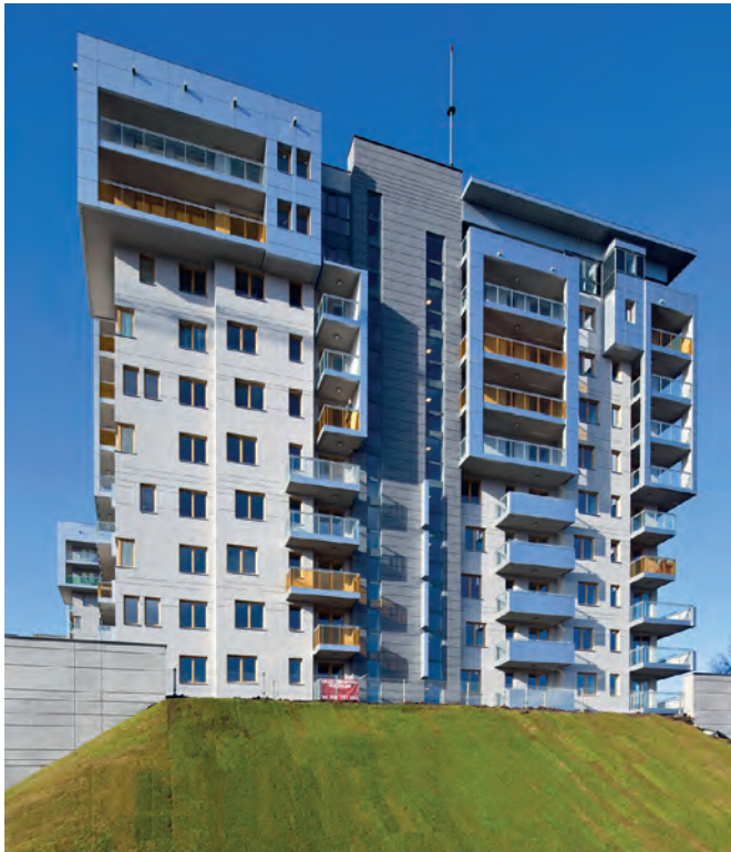
Thanks to the usage of precast elements, shorter construction times were reached, for example in the Osiedle City Park Project.
