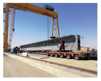
Due to the convenient location of the production yard, which is placed in the middle between the 2 furthest construction sites, the transport ways have been minimized to 20 km max.
