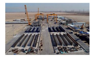
9 of the bridges are constructed with precast concrete elements, which are produced on a local precast yard by using of moulds from Tecnocom.
