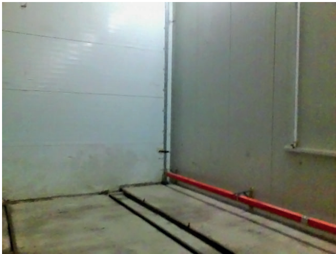
A corner of the curing chamber in which the concrete slab inside the chamber is exposed to the cold weather outside. The standing water may be seen in the picture while the ingress of cold, causing this standing water, is seen as purple on the thermal image.
