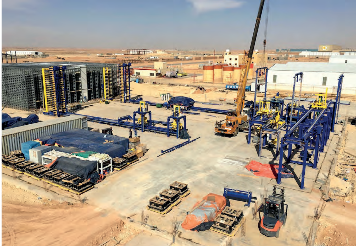
Assembly phase - The curing area with a rack plant from HS Anlagentechnik as well as the Masa finger car, elevator / lowerator and intermediate finger car are already in place.
