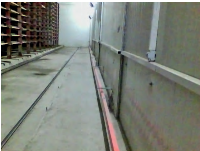
A typical transfer car area with an insulated exterior wall. Damp spots are seen throughout the area and the thermal image shows very well the coldness of the floor in the transfer car area due to poor air circulation. The dark purple spot and areas along the outside wall are indications of cold leaking into the chamber through the concrete floor.
