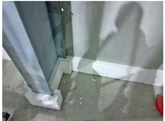
Insulation board is the solution for insulating the perimeter of the curing chamber after installing the rack and rails, but prior to placement of the screeded floor. All steel support beams for the production building must be insulated and isolated from the concrete inside the curing chamber. These steel columns are highly efficient thermal bridges and can cause numerous issues in the way of standing water.
