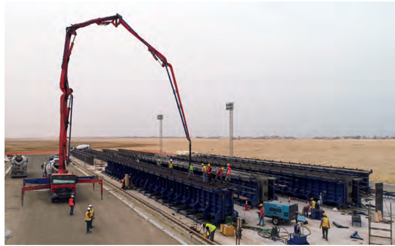
The moulds can produce elements with a length range from 40 - 45.5 m and can be adjusted to the required size.
