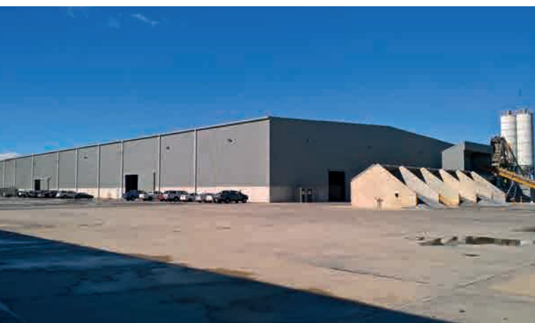
BGC Precast manufactures high quality architectural and structural wall panels to client's requirements in their modern factory in Kwinana. (Credits: BGC)
