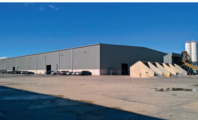
BGC Precast manufactures high quality architectural and structural wall panels to client's requirements in their modern factory in Kwinana. (Credits: BGC)
