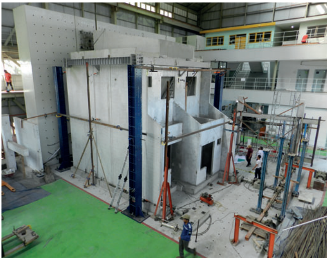
The property developer PT Modernland has made the topic of "earthquake-proof construction" a central aspect in the planning of its new precast concrete houses and overall projects.
