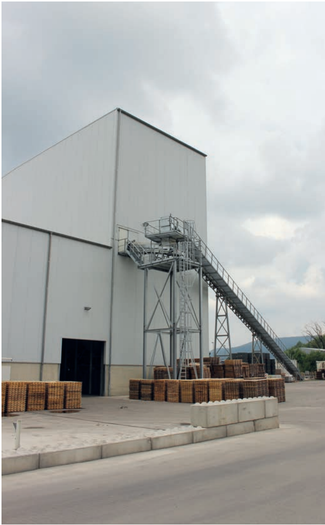
Facing concrete aggregates are transported to the silos by a steep conveyor belt.
