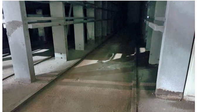
Typical effect of condensation: columns closer to the chamber's center are dry and free of corrosion while those located at the perimeter (right) have corroded at the bottom
