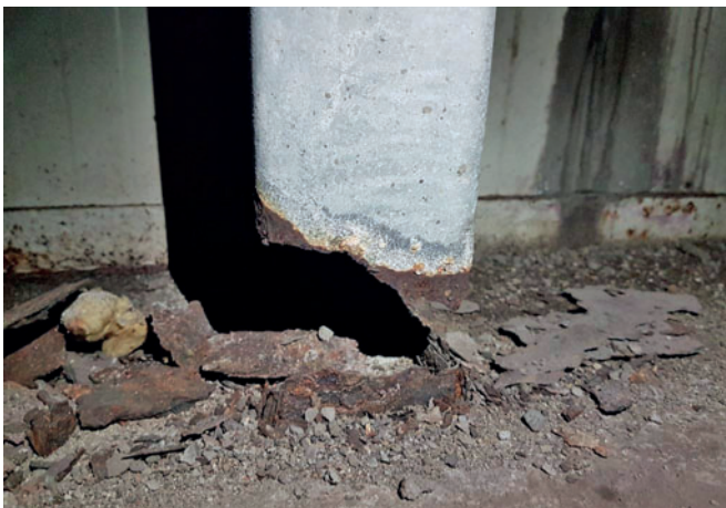
Column corroded due to condensation. This completely corroded lower column portion is only held in place by the rest of the rack system and requires immediate replacement
