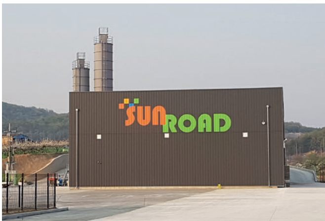
Sunroad's new concrete block plant
