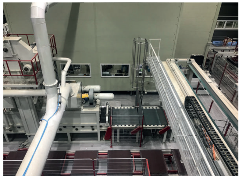
An inline blasting plant from Doogsan was integrated for further refinement.
