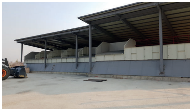
View of the aggregate silos
