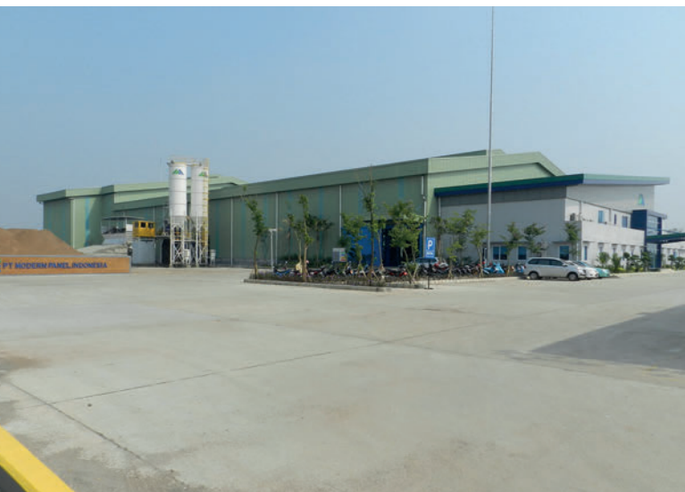
PT Modern Panel Indonesia recently opened its first precast plant in the new industrial estate of Cikande, Banten.
