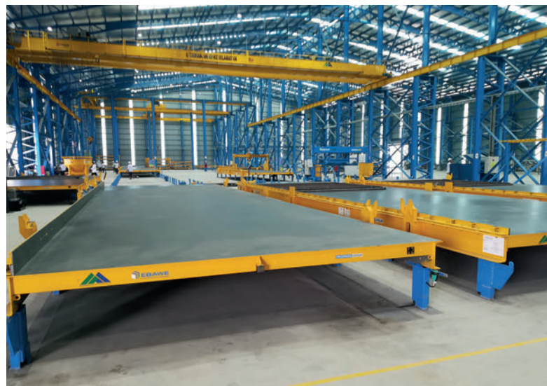
"In our new plant we have installed the very latest machine technology from Ebawe, which belongs to the Progress Group and is one of the leading suppliers of machines and solutions to the precast industry", says Hendy W. Budijanto, Managing Director Operations at PT Modern Panel Indonesia.
